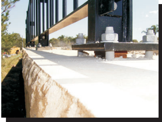
HAND RAIL FIXING
